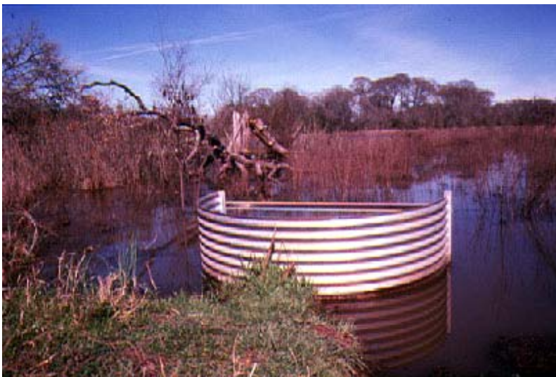
A water control structure built into a levee can create a shallow wetland that will benefit waterfowl and other wetland species.
